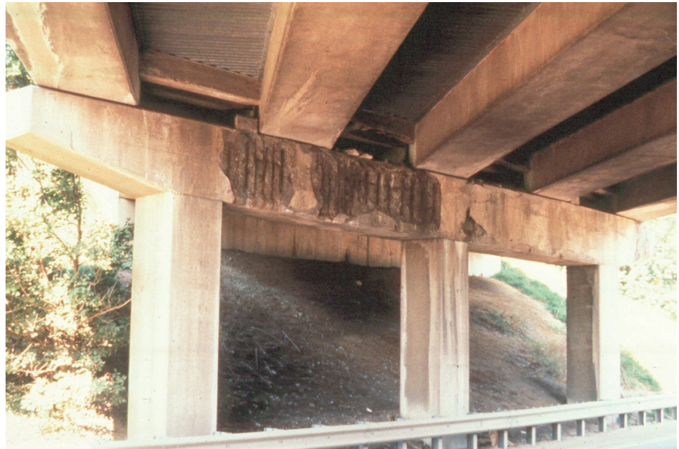
Figure 10.2.38 Severe Concrete Spalling on Bent Cap
