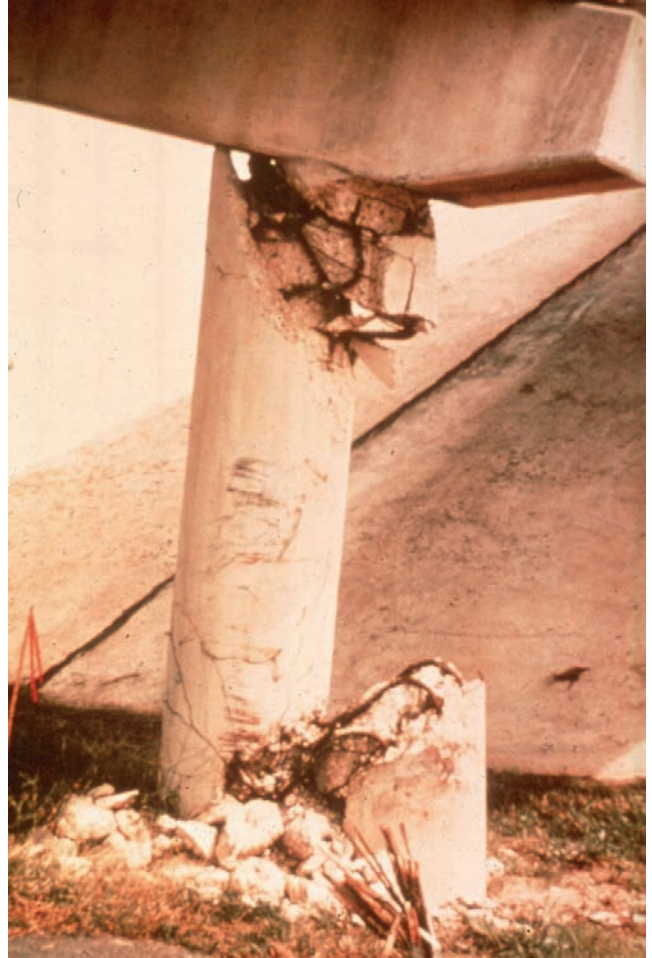
Figure 10.2.39 Collision Damage to Pier Column
