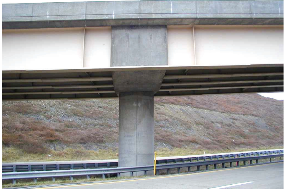
Figure 10.2.11 Integral Pier and Pier Cap
