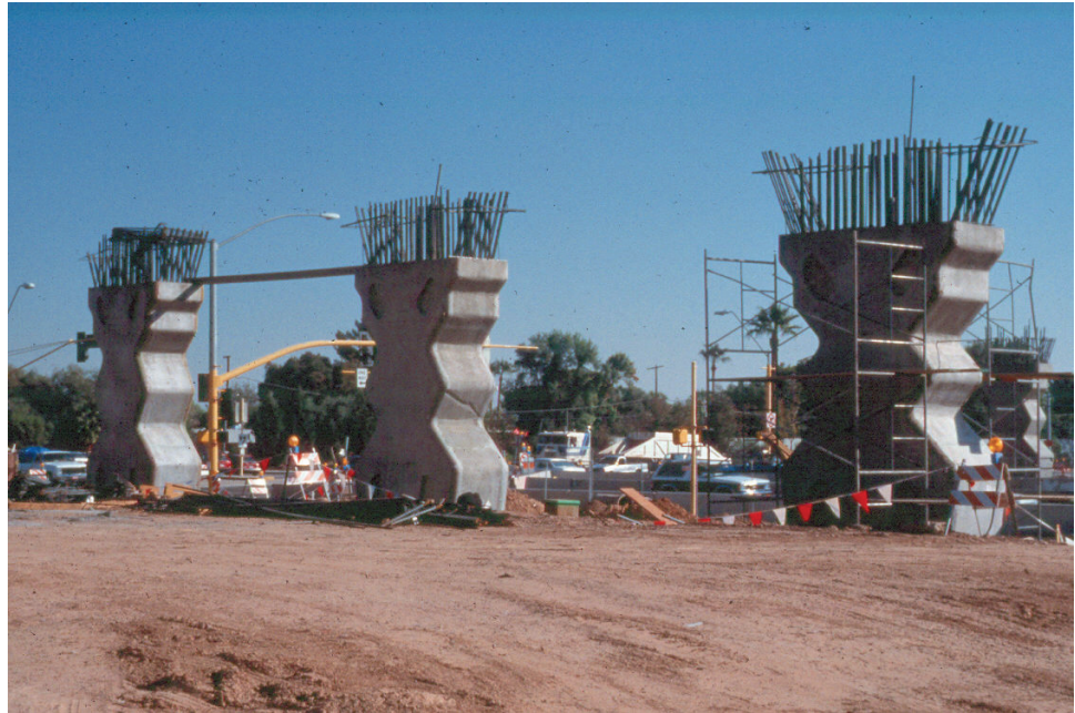
Figure 10.2.13 Reinforced Concrete Piers under Construction
