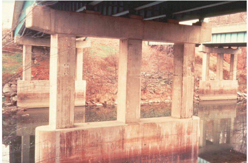
Figure 10.2.25 Collision Wall
