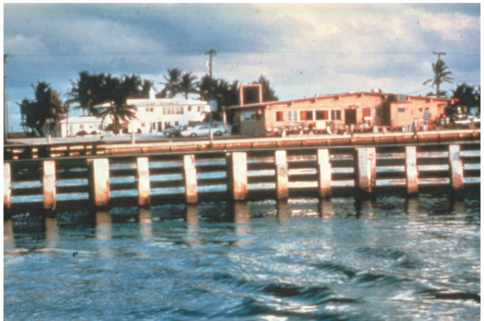
Figure 10.2.29 Fender System
