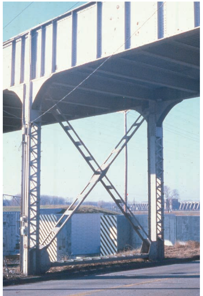
Figure 10.2.41 Corrosion and Debris at Steel Pile Bent
