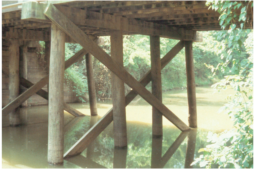
Figure 10.2.46 Timber Bent Columns in Water
