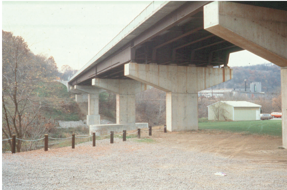
Figure 10.2.7 Cantilever Pier
