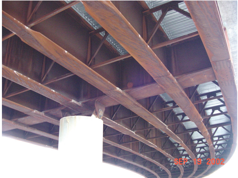
Figure 10.2.10 Integral Pier Cap
