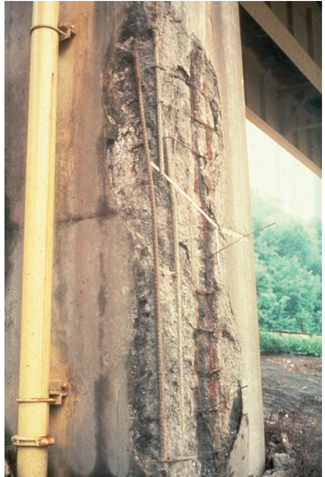
Figure 10.2.36 Concrete Deterioration due to Contaminated Drainage
