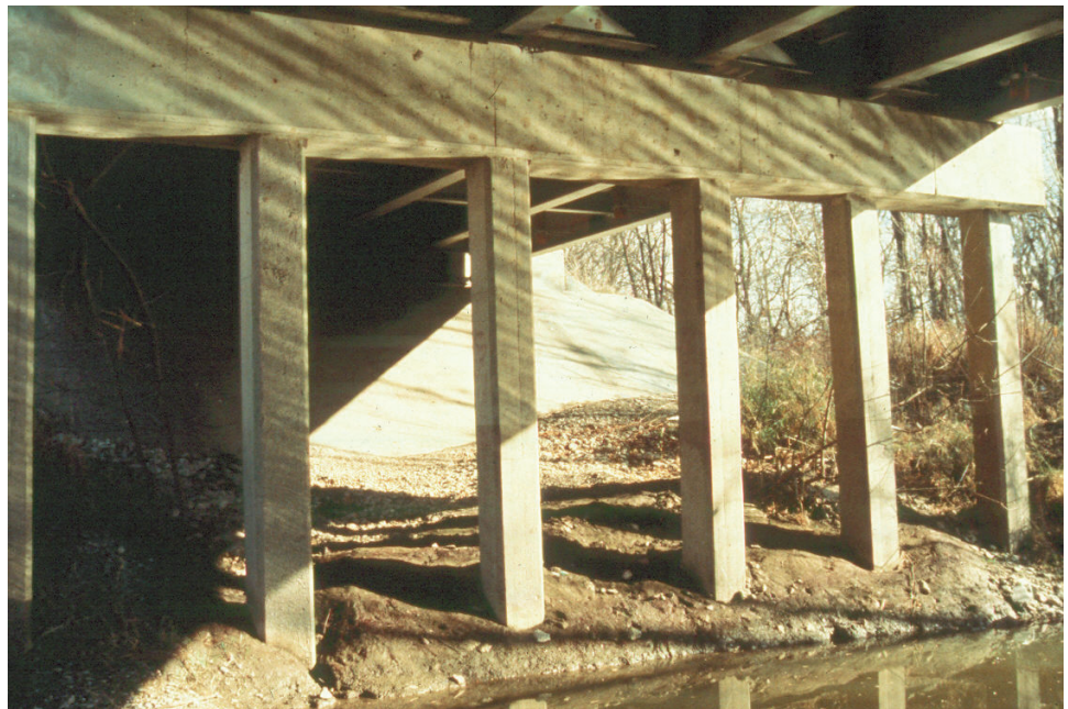
Figure 10.2.9 Concrete Pile Bent
