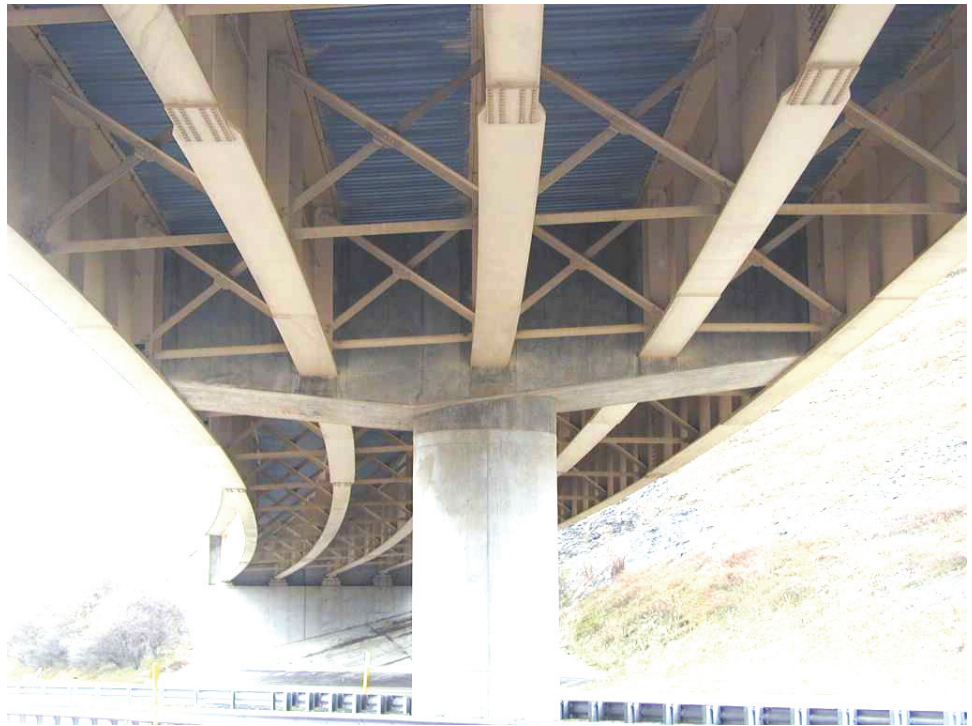
Figure 10.2.12 Integral Pier and Pier Cap
