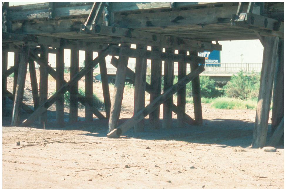
Figure 10.2.16 Timber Pile Bent
