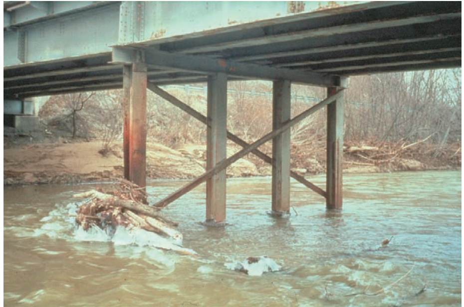
Figure 10.2.41 Corrosion and Debris at Steel Pile Bent
