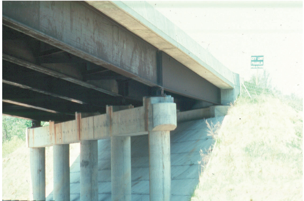
Figure 10.2.8 Column Bent or Open Bent
