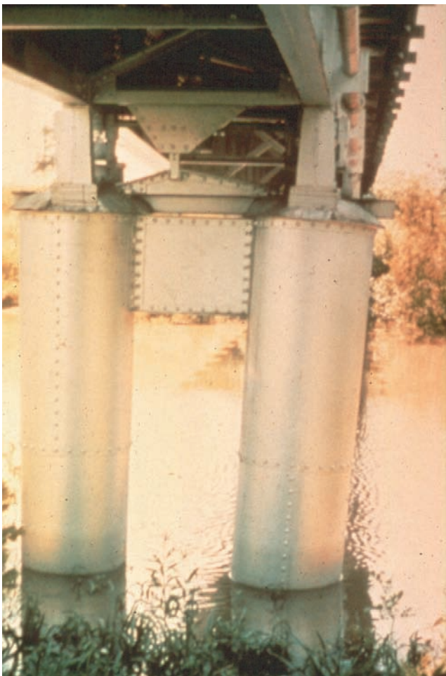
Figure 10.2.35 Tipping of Bent due to Scour/Undermining
