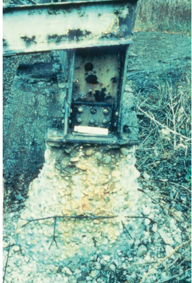
Figure 10.2.40 Deterioration of Concrete Pedestal Supporting Steel Column
