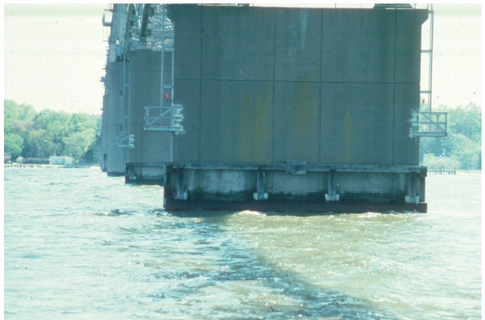
Figure 10.2.54 Steel Fender
