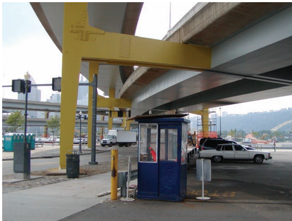
Figure 10.2.52 Fracture Critical Steel Bent
